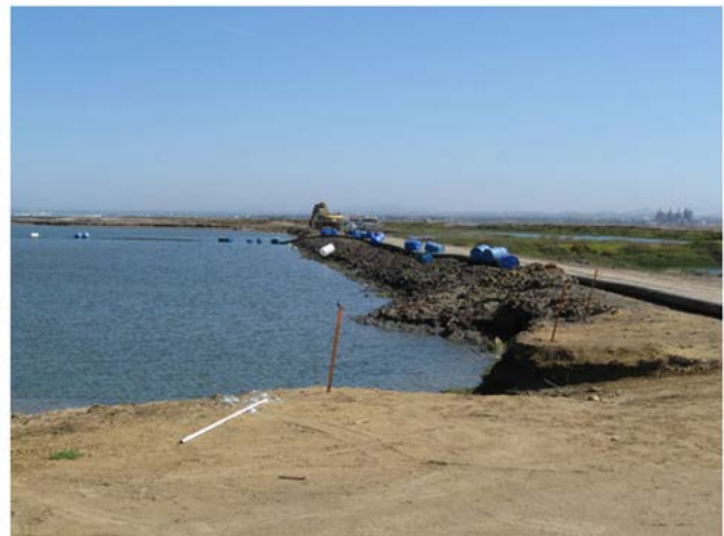
Salt Ponds under construction to allow tidal water flow
